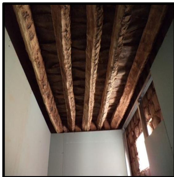
Figure 9: Image showing the construction of the toilet adjacent to the lobby.
