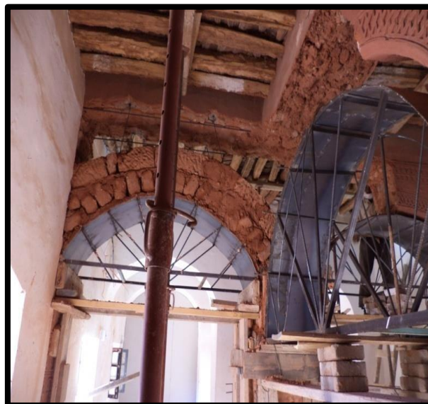
Figure 16: Image showing the restoration process of the arch support.
