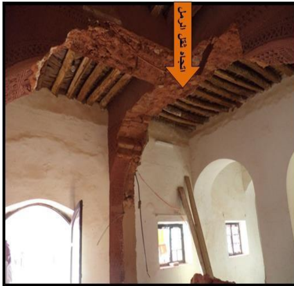
Figure 15: Image showing the collapse of the support for the three arches due to the removal of the wall.
