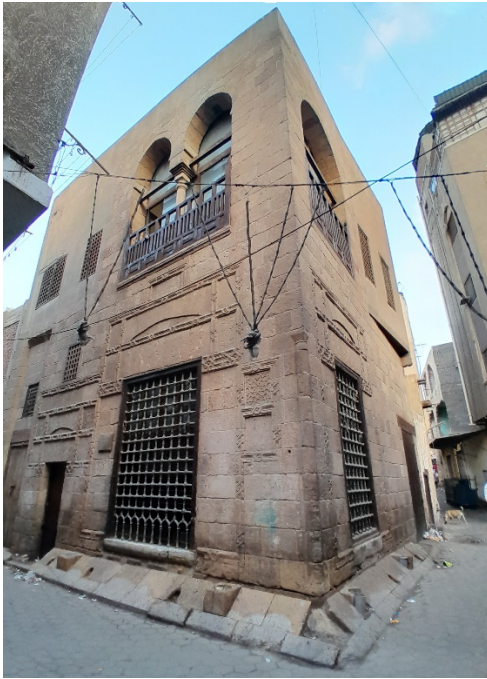
Figure 3. The exterior elevations after relocation
