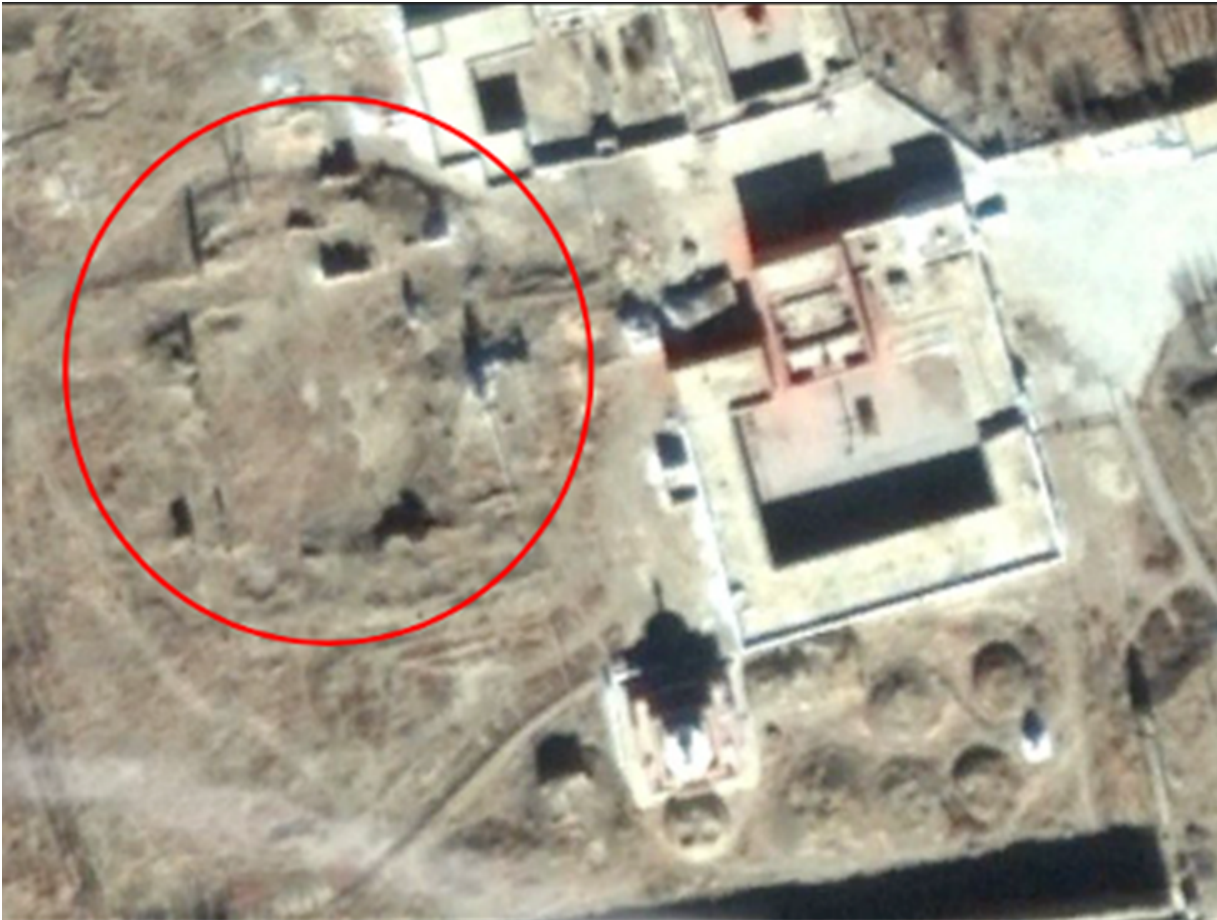
Figure 18. New Parkhang and nearby demolition remains (Google Earth 2011).
