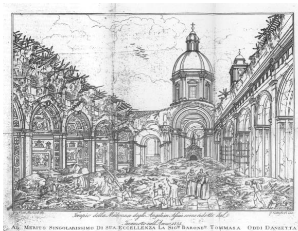
Figure 3: The collapse of the Basilica's nave after the 1832 earthquake [3].
