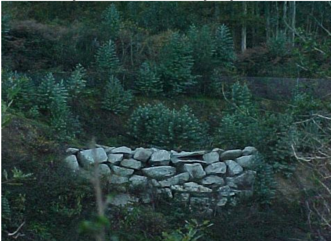
Fig.2. Muro escollera (Stone wall Hard-engineering Technics)
