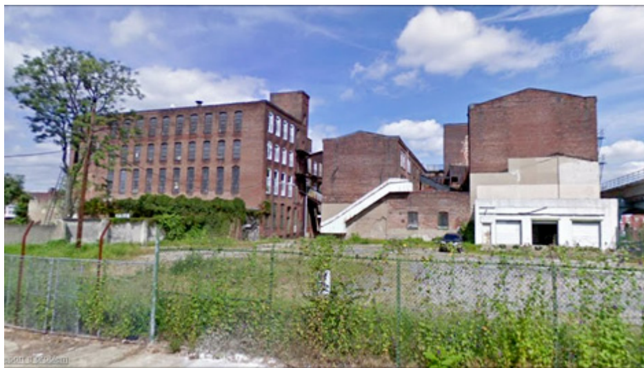
The Quaker City Dye Works complex before work began.
