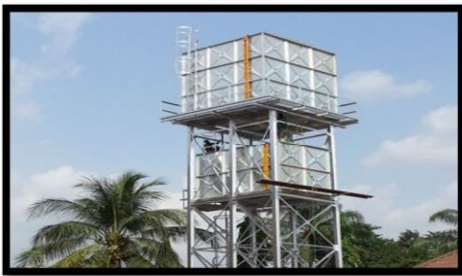
Figure 18: Overhead Steel Water Tanks
