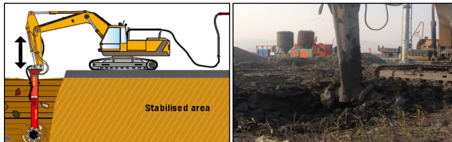
Fig 1. In-situ curing technology
