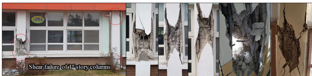
Figure 2. Shear Failures on Short Column effect
