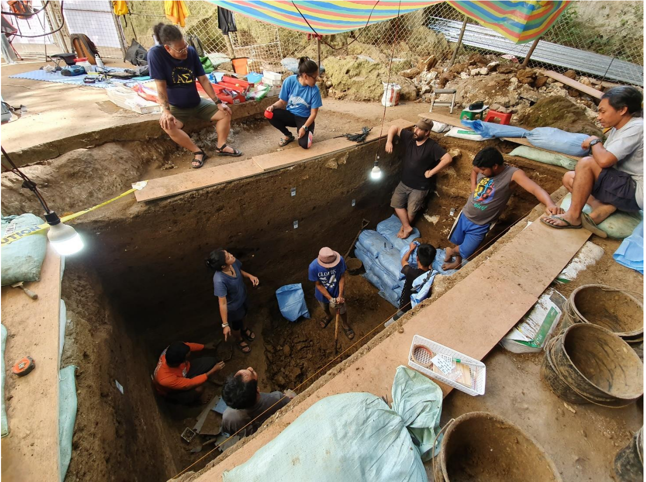
Fig. 26 Upon reaching around two meters below surface, the two squares were combined into one four by two-meter trench and excavated simultaneously. The trench's edges were lined with plywood beams to prevent loose soil from collapsing. Sacks full of sieved sediments were placed in the western portion to serve as an entry and exit point. Archaeologists were encouraged to enter the trench barefoot as a precautionary measure for unexcavated delicate artefacts, if any. Source: KD Tantuico, 28 February 2020.
