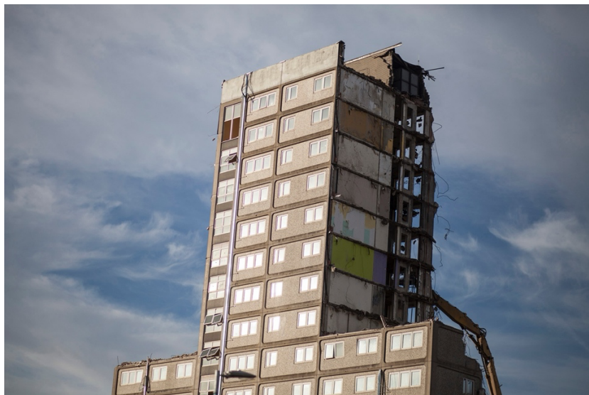
Figure 8. Demolition of Apple Tree Court in Pendleton, Greater Manchester. November 25 th 2014.
