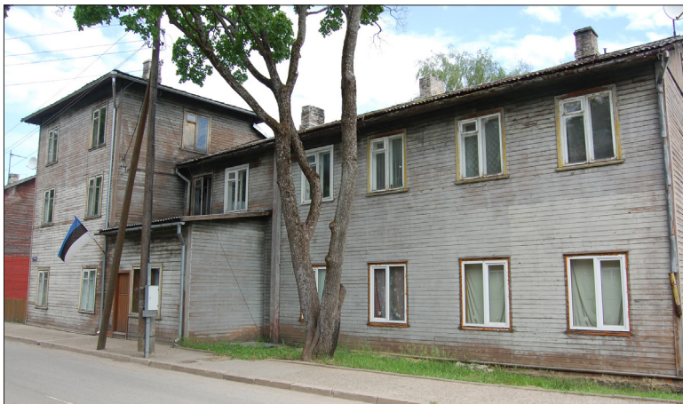
Figure 2: E. Enno 2 apartment building before demolition
