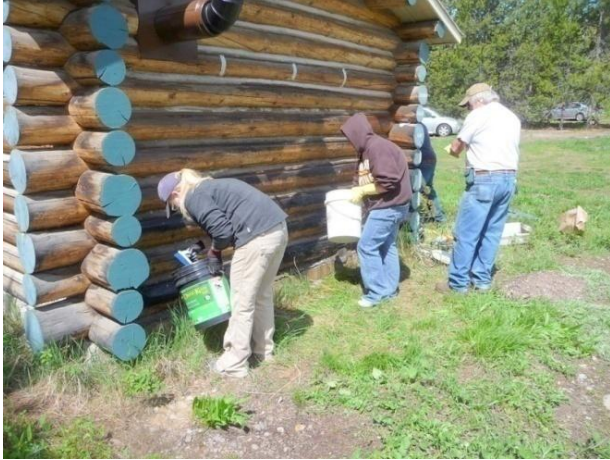
Figure 3. Students prepare a log wall for testing to compare the effects of different log cleaning techniques. (Mary Humstone, 2011)
