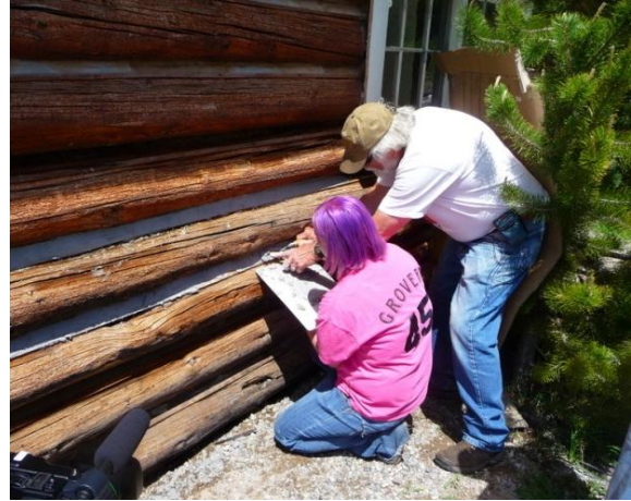
Figure 5. Harrison Goodall shows student Cassie Loveland how to apply daubing to the logs of the boathouse at AMK Ranch. (Mary Humstone, 2011)
