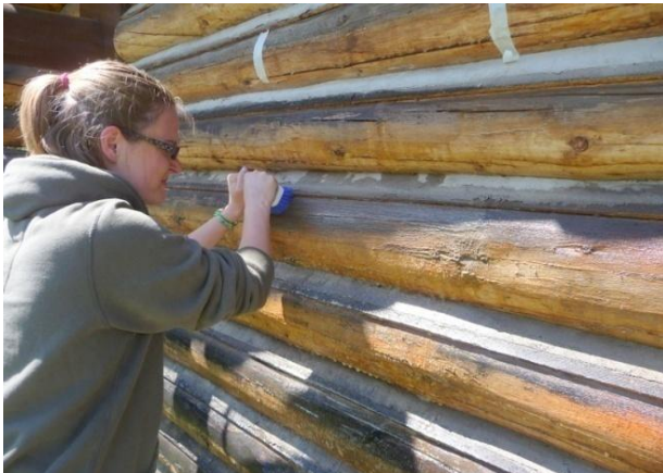
Figure 4. UW student Andrea Lewis cleans logs with abrasive brush after applying a cleaning solution. (Mary Humstone, 2011)
