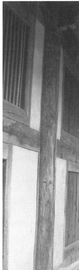
A view along the side of one of the storage buildings.
