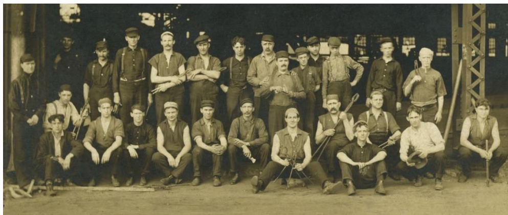
Figure 4. 1906. Rolling Mill Crew . Photograph. Pittsburgh, PA. Jones & Laughlin Steel Corporation Collection Photographs, 1864-1953, MSP 33, Library and Archives Division, Senator John Heinz History Center. MSP33.B005.F24.I02. Available online: https://historicpittsburgh.org/islandora/object/pitt%3AMSP33.B005.F24.I02 (accessed on 27 September 2024).
