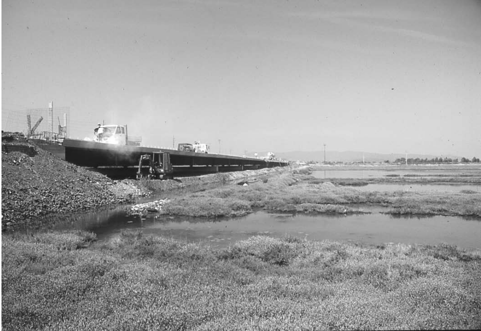
Fig. 1: The viaduct under construction (2002), seen from the 'Orti' brackish marsh. Piombino, Province of Livorno, Tuscany, Italy.
