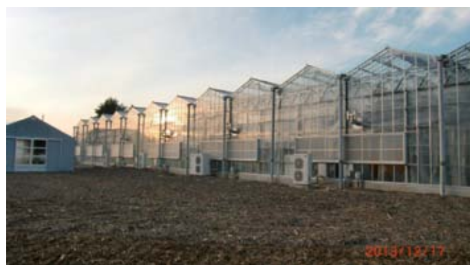
Fig. 5 - A multi-span type glasshouse with small roofs constructed in Tsukuba City, Ibaraki Prefecture.
