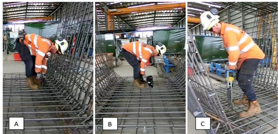
Figure 3 Use of the conventional pincer-cutter (A), power tying tool (B) and long handled stapler tool (C) at ground level
