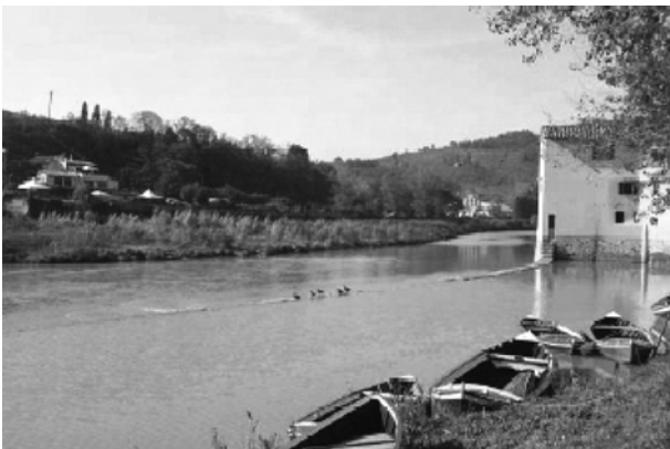
Fig. 6 - Modern view of the Arno River upstream of Florence. Former gualchiere are today converted into residential buildings. These buildings protruded into the channel, significantly narrowing the hydraulic section.
