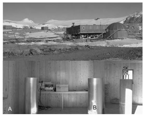
Fig. 1a,b. Geomagnetic observatory at Mario Zucchelli Station: a) variometer shelter; b) absolute measurement shelter.
