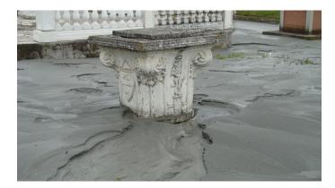
**Figure 2.** Example of sand ejection from a large-diameter water well at the base of the levee associated with an abandoned reach of the Reno River (San Carlo-Sant'Agostino road).
