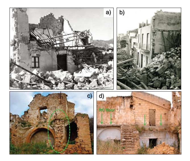
**Figure 4.** Example of buildings with vulnerability Class A. Collapse of structures built with squared blocks of soft calcarenites assembled with little mortar: a) Poggioreale; b) Santa Margherita (photos by *L'Ora*, 1968). c) Santa Margherita, masonry with very irregular stones, assembled with very poor mortar and d) interventions of elevation with RC slab floors and heavy blocks of calcarenites above a weak masonry (when not specified, photos are by the authors of this study).
