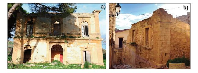
**Figure 6.** a) Poggioreale, a solid masonry structure with massive stone (Class C) still standing after fifty years of abandonment; b) Salemi, example of a vulnerability Class B building with massive cornerstones; note that the upper part of the house was demolished to make safe access to the street.
