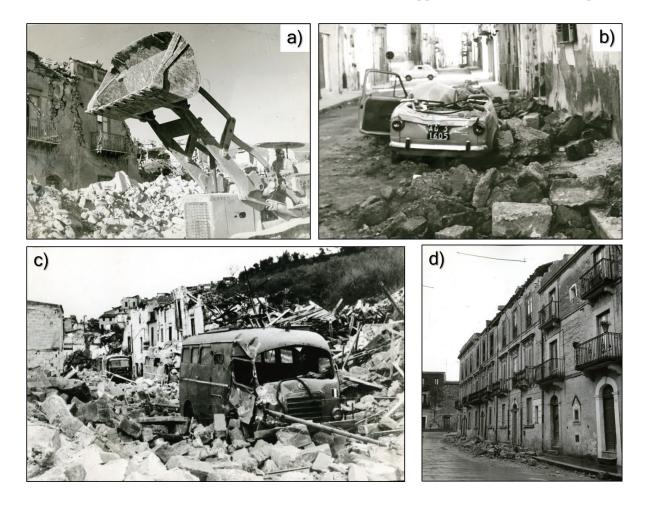
**Figure 8.** a) Salaparuta, ruins were raised to the ground by bulldozers; b) Menfi, partial collapses meant highly dangerous situations but luckily there were no victims; c) Gibellina, the last collapses due to the 25 January earthquake also led to casualties, including deaths in the rescue teams; d) Salemi, collapse of the eaves and damage to the upper part of the edifice (photos by *L'Ora*, 1968).
