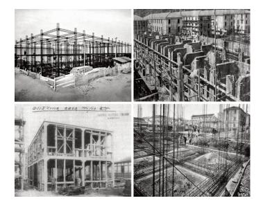
FIGURE 2. Construction systems for "anti-seismic" structures permitted after 1908 Messina earthquake: frames of steel (1909 et seq.); reinforced masonry (from 1912 to 1924); reinforced concrete frames with diagonal bracings (1909); frames in reinforced concrete with rigid knots (1909 and then since 1924).
