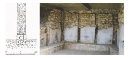
FIGURE 1. On the left reconstruction of a wall in Tylissos with stone socle, timber frame and rubble filled interior [Shaw, 1971]; on the right timber traces in the Hagia Triada villa [Tsakanika and Theohari, 2009].
