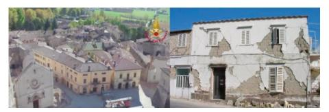
FIGURE 5. Example of damage occurring in: a) Norcia, after the 2016 earthquake and b) Ischia, after the 2017 earthquake.
