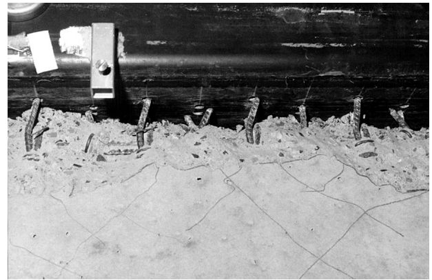
FIGURE 13. Detail HSW7 after test.
