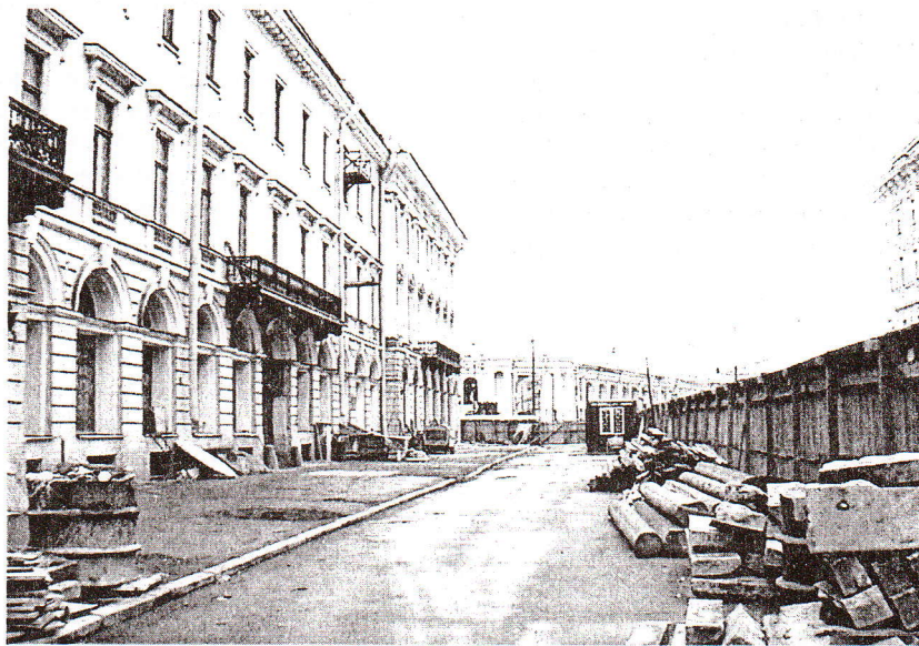
Fig. 6: Promstroibank St Petersburg, Russia – north-west facade
