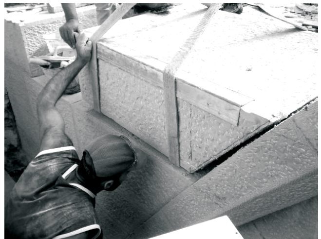
Fig. 18: Assembling the spandrel stones
