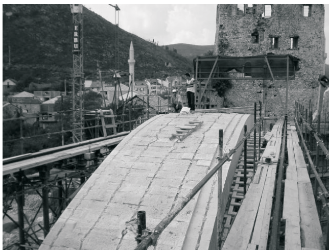
Fig. 12: Load bearing arch completed
