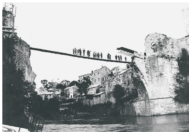
Fig. 3: Destroyed bridge – south elevation
