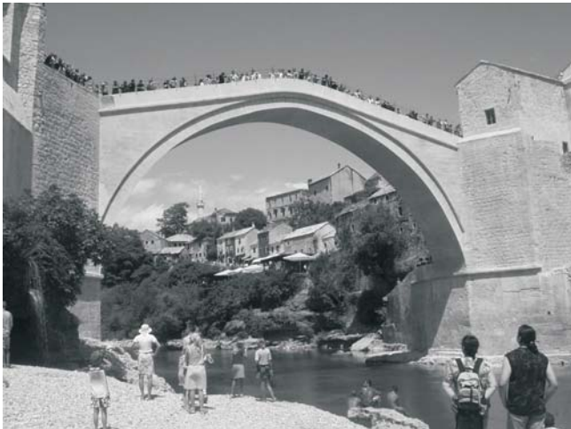
Fig. 29: New Old Bridge today
