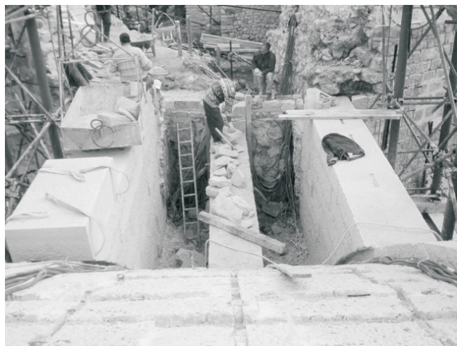
Fig. 20: Assembling the upper cornice
