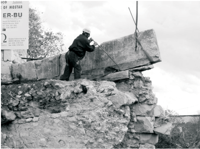
Fig. 7: Dismantling the remnants of the bridge on the south east side
