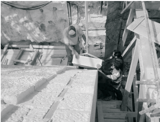
Fig. 16: Assembling the cornices
