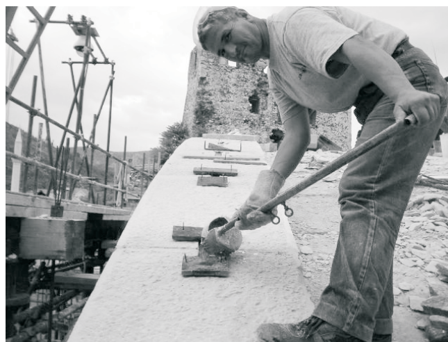
Fig. 24: Pouring the lead
