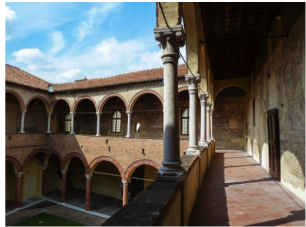
FIGURE 1. Inner yard of Casa Romei.
