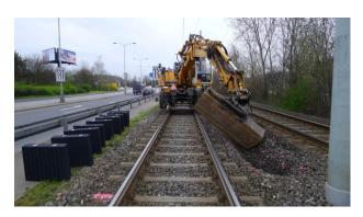
FIGURE 5. Groove excavation for mounting MNAS using the MHS two-way excavator.
