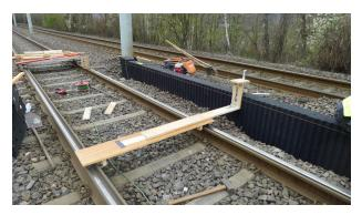
FIGURE 7. Checking the screen distance and height from the rail axis and TR.
