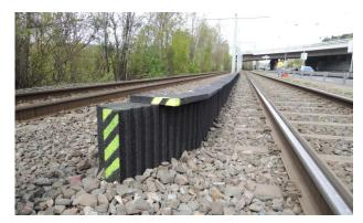
FIGURE 10. Municipal Noise-absorbing Screen after modification.
