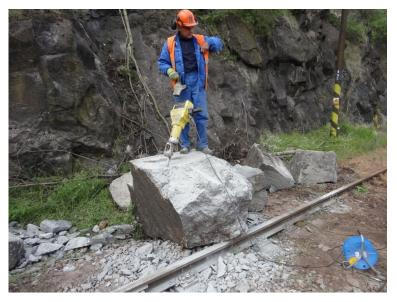
FIGURE 3. Fallen rock block after partial disintegration.
