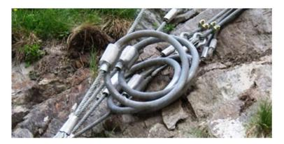
FIGURE 7. Detail of a loop-type breaking element (energy absorber) of the dynamic barrier.
