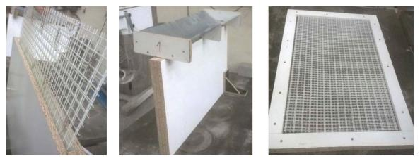
FIGURE 4. Formwork for TRLC slabs with 3D glass textile.
