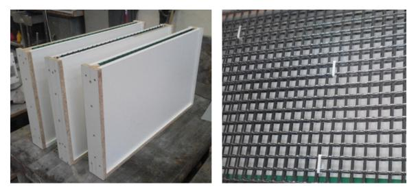
FIGURE 3. Formwork for TRLC slabs with 2D carbon textile.
