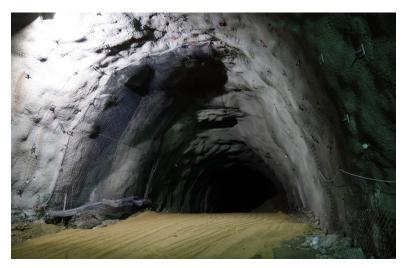
FIGURE 4. The collapse 2 mouth protection by the high-tensile steel mesh.
