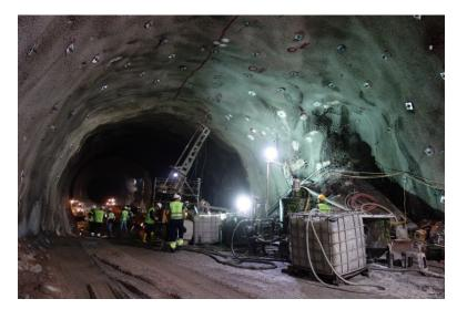
FIGURE 5. Grouting of the collapse 3, its mouth situated behind a barrel with grout.
