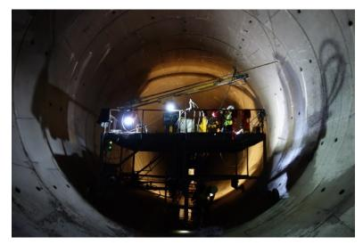
FIGURE 6. Core drilling in the TBM tunnel.
