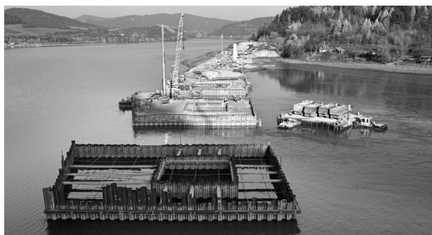
FIGURE 6. A heavy stone backfilling
