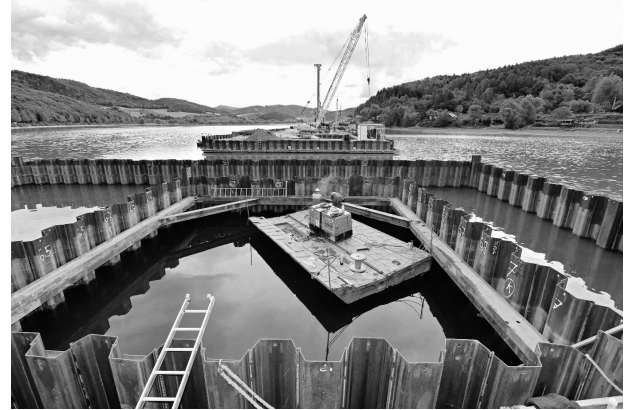
FIGURE 4. Mounting the spacer frame in the sump
