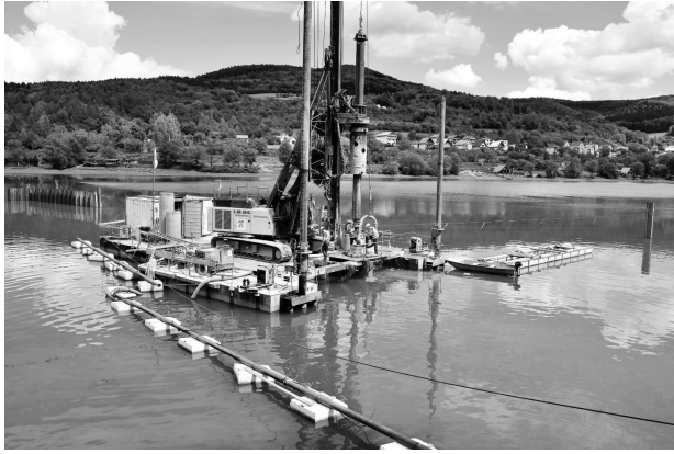
FIGURE 2. Realization of piles from pontoon
