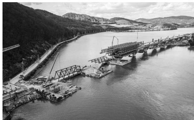
FIGURE 1. New railway bridge over the Nosicka Dam during construction
