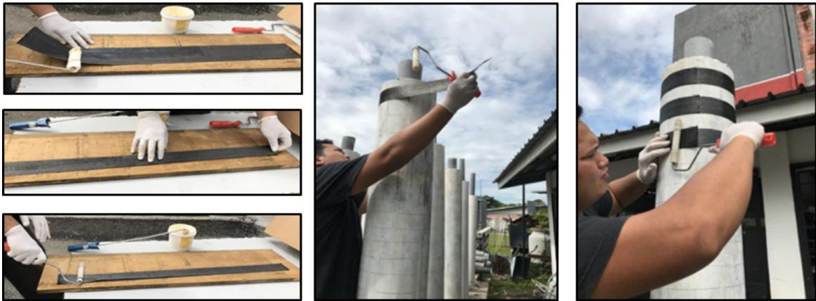
FIGURE 2. Partial CFRP Installation; (a) Adhesive Application on CFRP Strip (b) CFRP Strip Installation on Concrete Surface.
