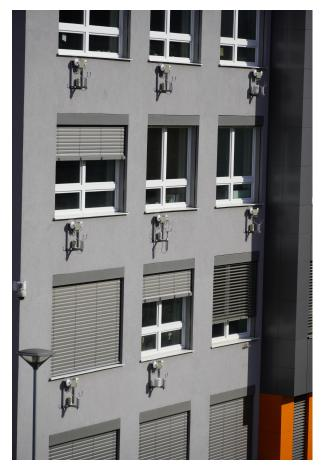
FIGURE 2. Meteo-stations located on the west facade of the Research Centre.
