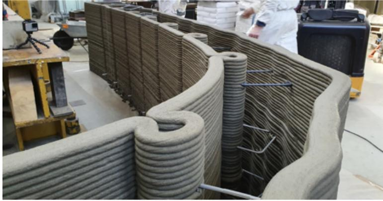
FIGURE 7. Construction of the wall during the printing.
