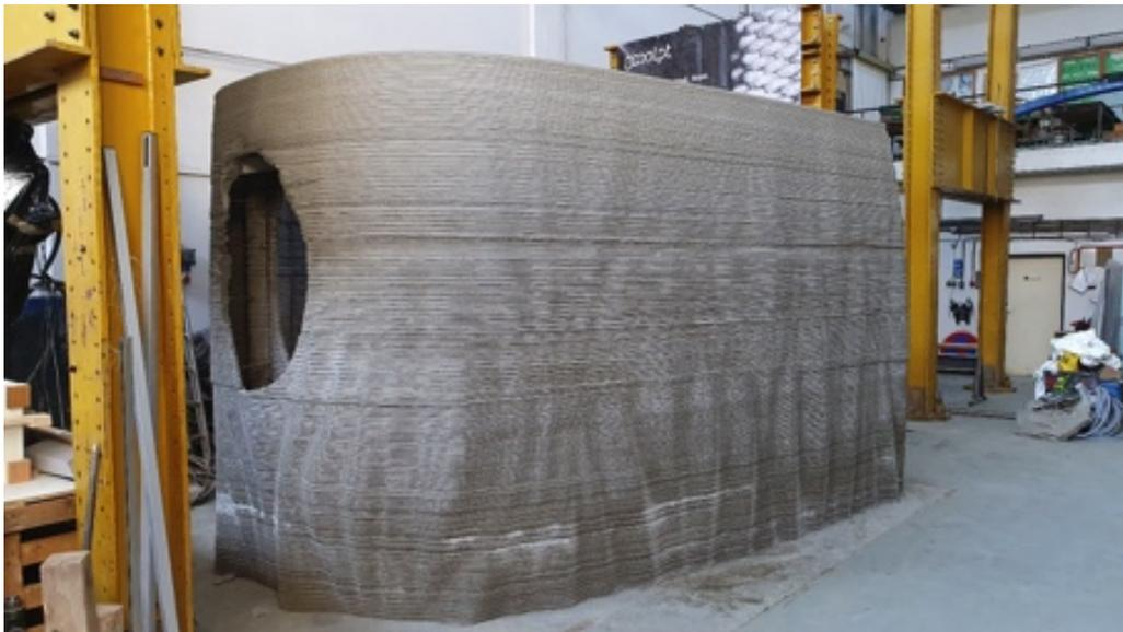
FIGURE 6. Printed segment of the PRVOK.
