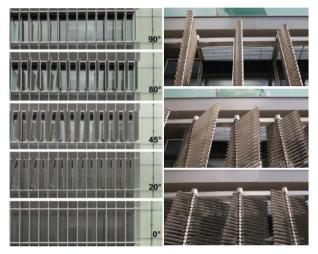
Figure 10. Different states of the sun-shading kinetic system
