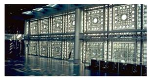
Figure 7. Interior shots of Institut Monde Arabe shows the sensitive diaphragms which regulate the amount of daylight entering the building
