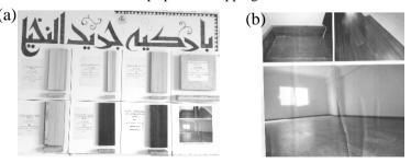
Figure 10. Photographs of (a) Palm frond parquet Flooring (b) Room with Palm frond parquet Flooring covered with a layer of beech wood Source:[Egyptian Association for self-development of local communities, Egypt, researcher photo]
