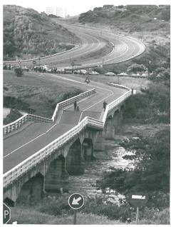
Figure 3. Caissons failure due to bed erosion (Frankipile, 2008)
