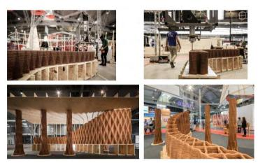
Figure 15. Robotos driven by cables & drones have helped in 3D printing using clay in printing large scale construction
