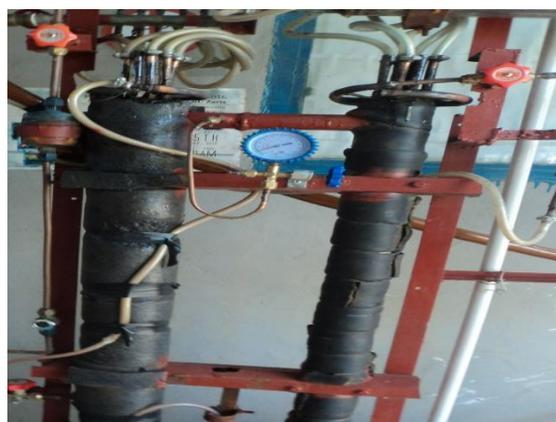
Figure 3: Section of the absorption chiller
