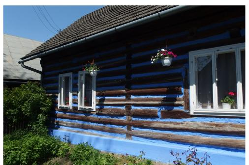
Figure 8 - Detail of blue painted gaps between wooden framework beams and blue primed plinth in Tylmanowa village (photo by Justyna Tarajko-Kowalska 2015)
