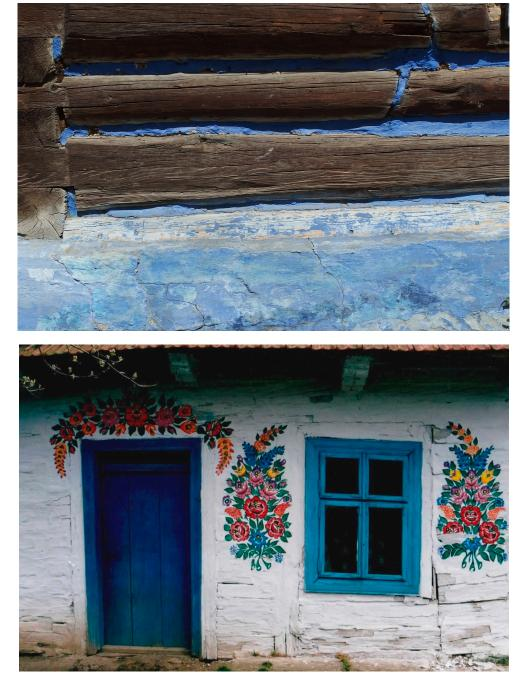
Figure 2 - Detail of blue painted gaps between raw wooden framework beams and blue primed plinth of the traditional cottage in Tylmanowa village (photo by Justyna Tarajko-Kowalska 2015)
