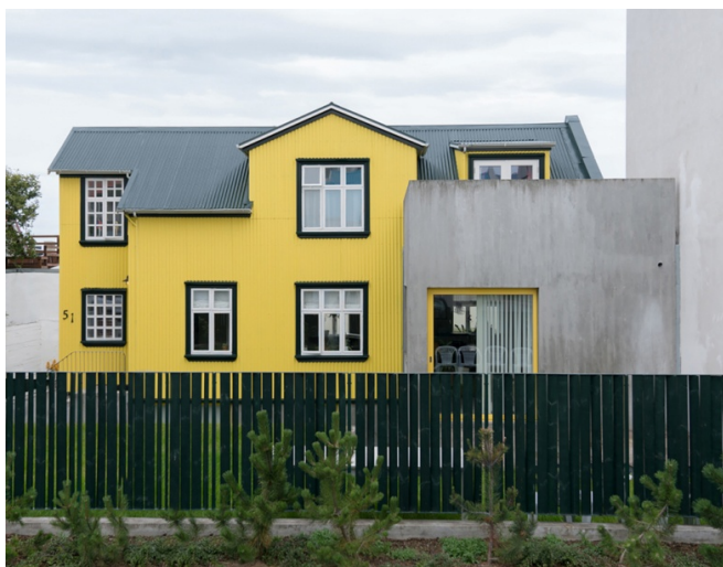
Fig.4. Façade of Njálsgata House in Reykjavik on Iceland selected for the presentation of colors in survey.
