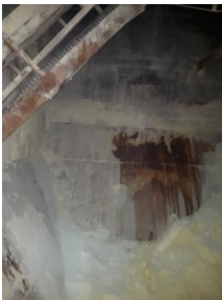
Figure 1: View from the sulphur silo manway
