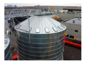
Figure 5. Vent panels installed on the top of a silo.
