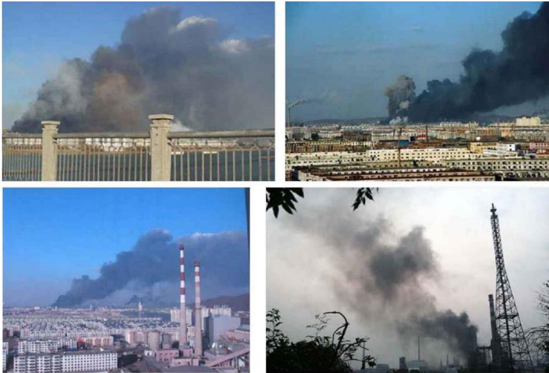
Figure 2: Leak site proliferation instances.
