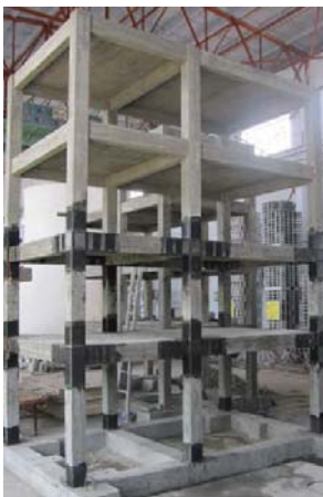
Figure 1: The frame model after CFRP reinforcement
