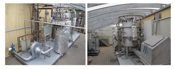
*Figure 1: Autothermal gasification technology: a) gas cleaning devices - hot filter, gas cooling and exhaust fan; b) fuel bin and fuel transport into autothermal gasifier.*
