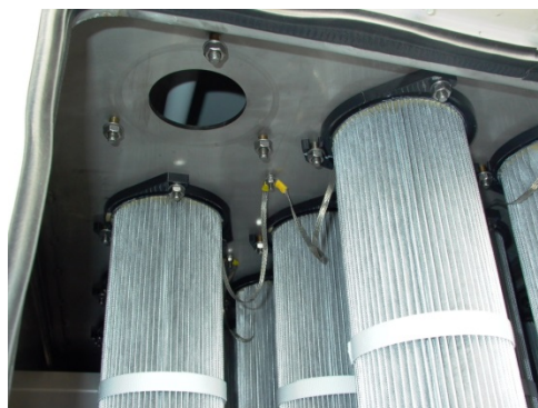
Figure 7: Cartridges - Mount on the raw gas side
