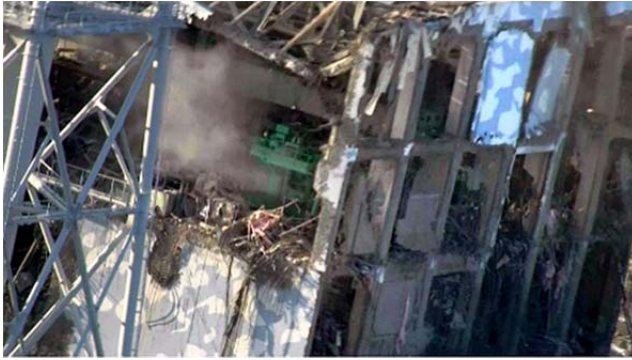
Figure 2. A plume of white smoke rises from around SFP of Unit 4 after the hydrogen explosion (Taken by TEPCO on 16 Mar. 2011)
