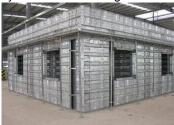
Figure 1: The aluminum alloy formwork
