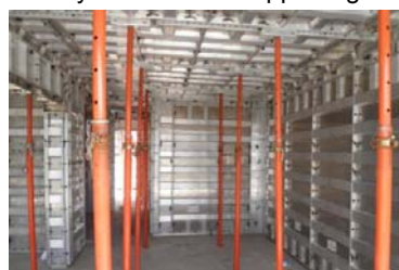
Figure 2: The aluminum alloy formwork in supporting structure
